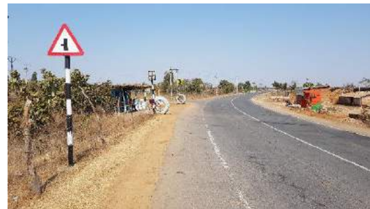
Cross Road at Km. 48+500
