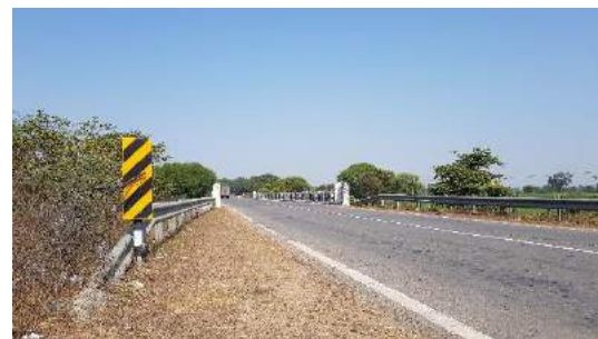
OH marker board before the Head wall of Box MJB at km.41+600
