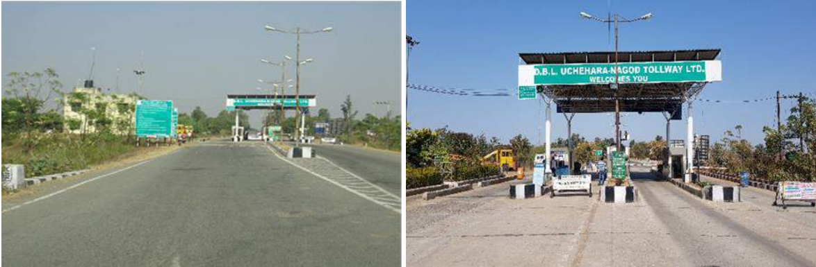
Figure 2.4: Toll Plaza at Km. 47+950
