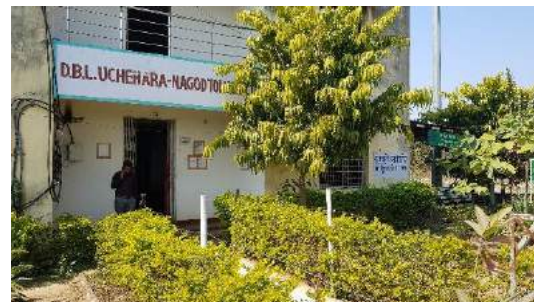
Toll Building at 47+950
