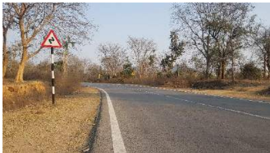
S-curve ahead Km. 85+300
